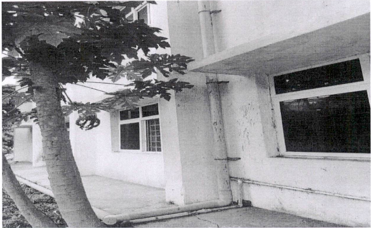
Geotagged photo of pipe distribution from overhead tank to rain water storage
